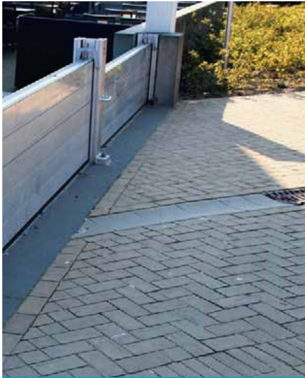
Abb. 53: mobile Flutmauer; Quelle: Embeki / stock.adobe.com
