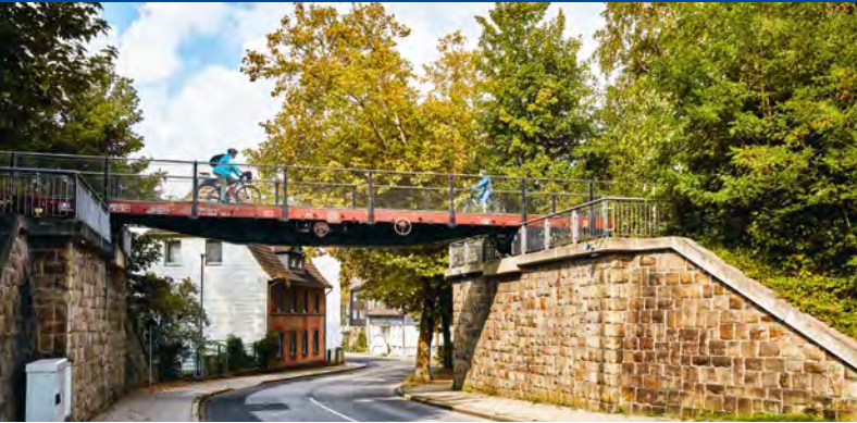
Waggonbrücke in Heiligenhaus
